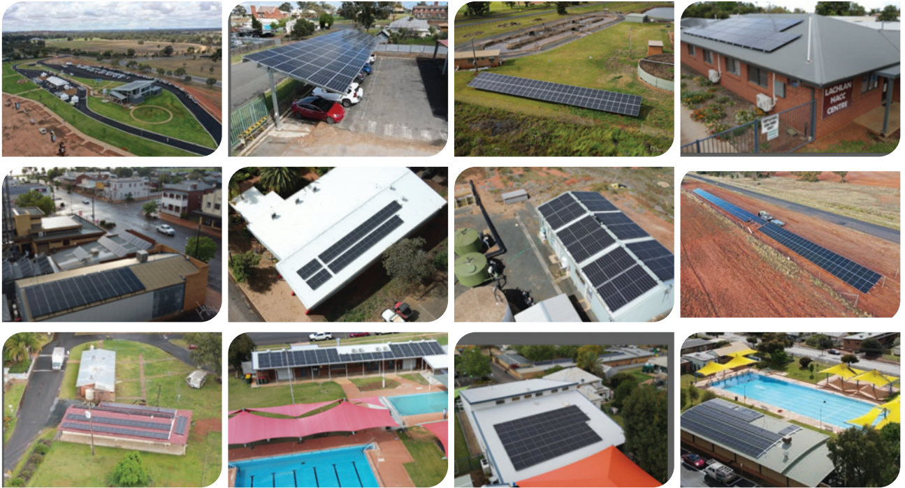
Figure 3: 660kW Solar PV Portfolio
