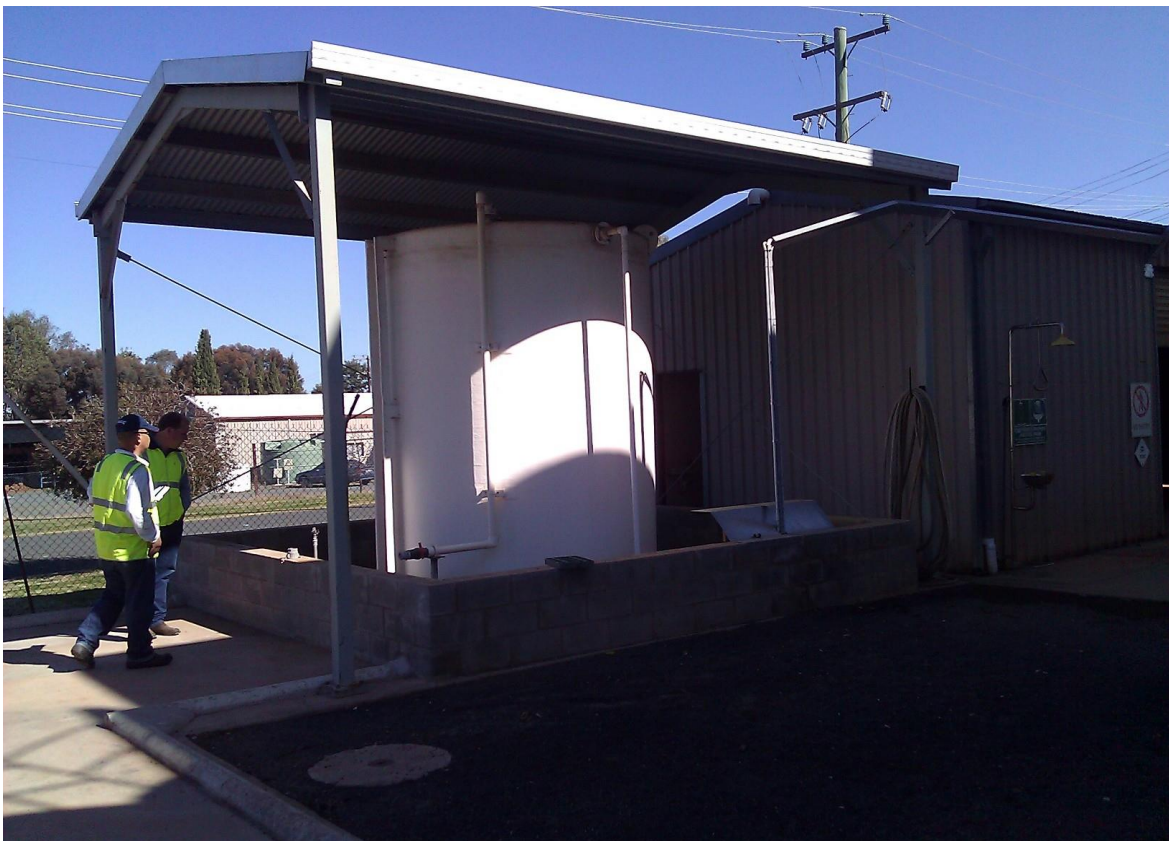
Figure 4.2 - Photo ACH Tank and Bund
