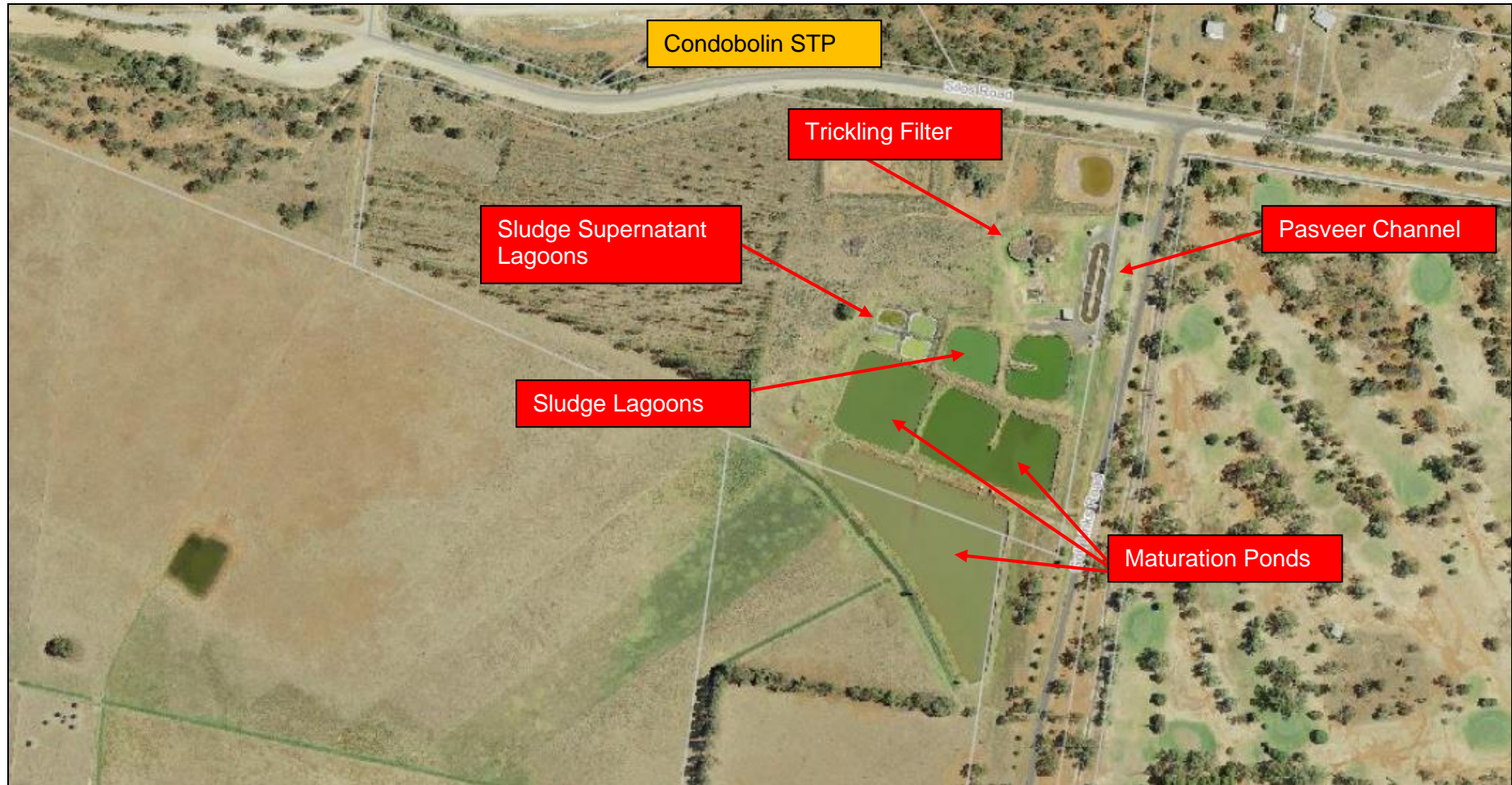
Figure 10.1 - STP Aerial Photo
