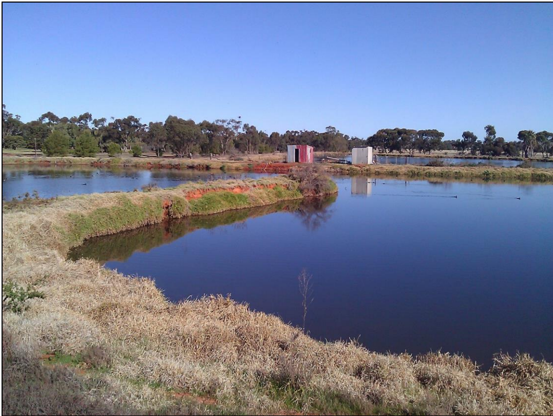
Figure 4.1 - Photo STP Maturation Ponds
