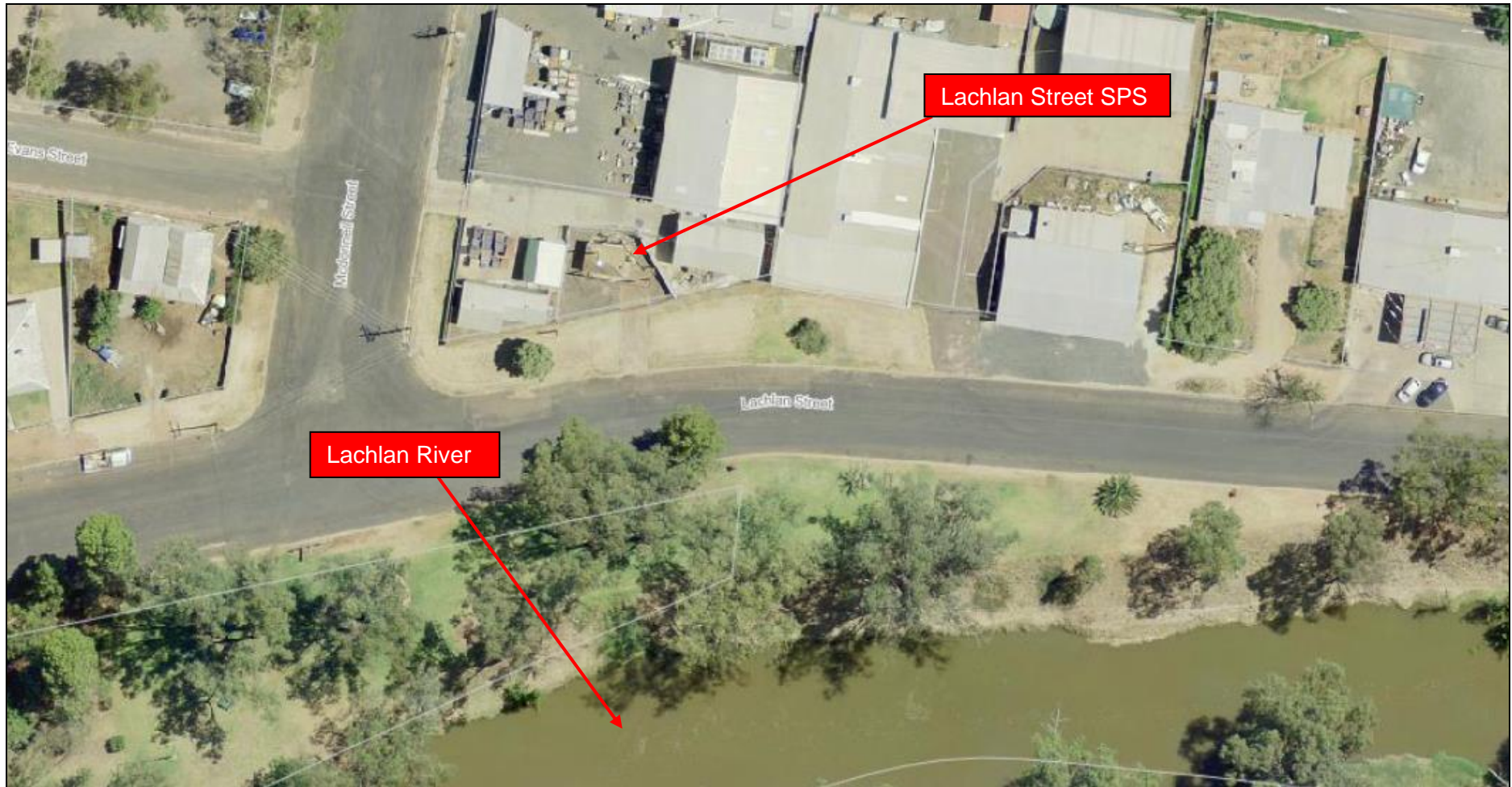
Figure 10.4 - Aerial Photo Lachlan Street SPS
