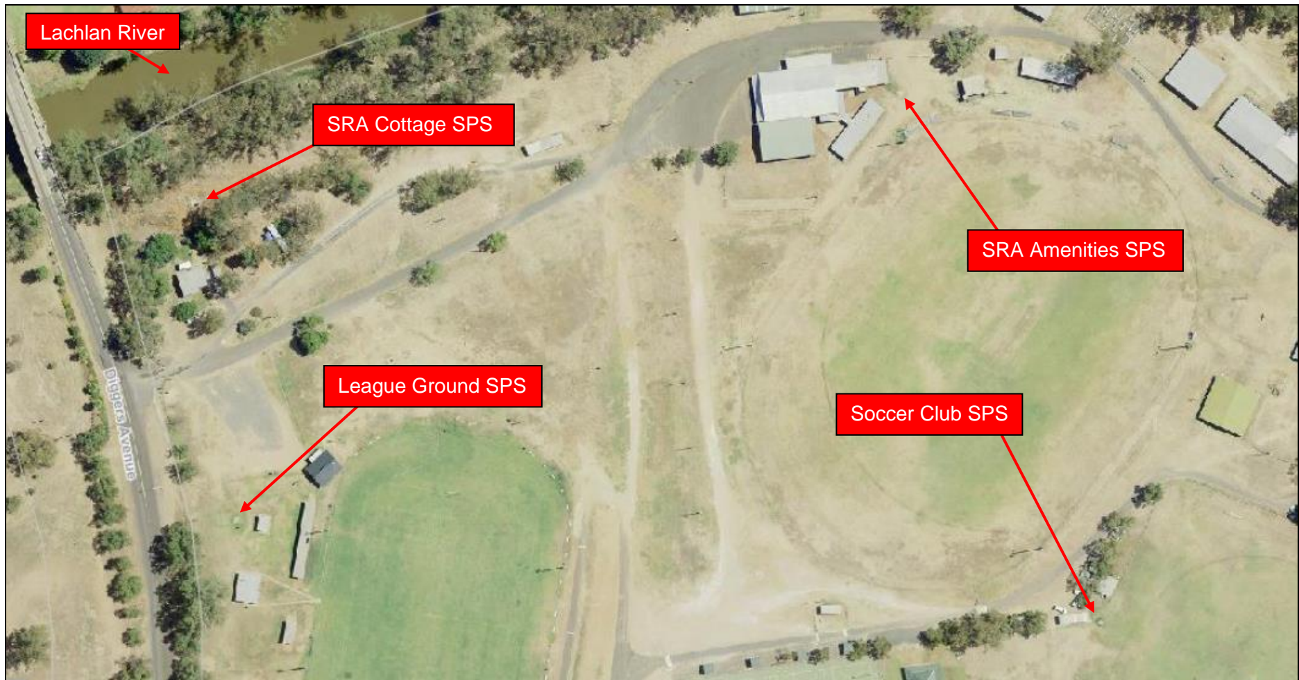
Figure 10.5 - Aerial Photo SRA Cottage SPS and Substations
