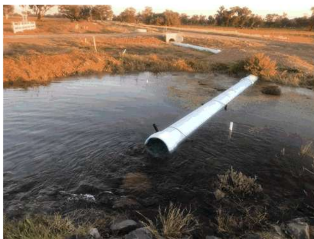
Discharge and Sampling location adj. BH 1
